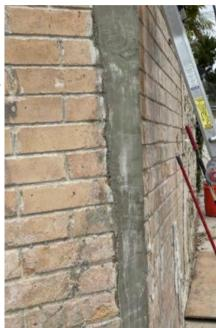
The large void in the broken corner joint was filled with a non-compressible hydraulic cement prior to the installation of the CFRP. To ensure a a flat and even profile was met beneath the carbon fiber, each mortar joint was filled flush to allow for the SRS-600 Unidirectional carbon fiber to be securely wrapped around each side to provide global strengthening of the corner.
