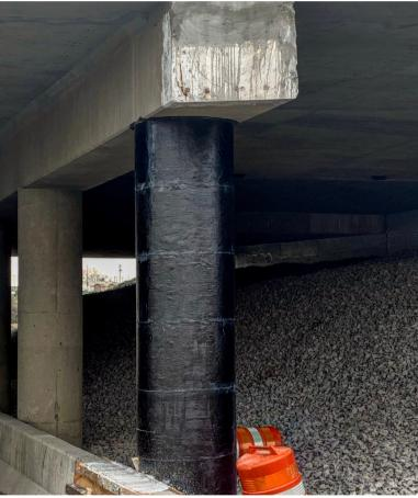
On columns where both flexural and confinement strengthening is required, an applicable design with either unidirectional or bidirectional fabric can be applied to provide increased capacities for the component.
