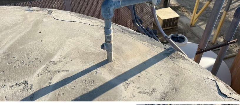
There was a fair amount of cracking on the outer perimeter of the lids as well as around the opening to the tanks. Upon completing the inspection on the tanks, a plan was put together to repair the concrete and confine the entire outside edge of the tanks as well as the tank openings with SRS-660BI.
