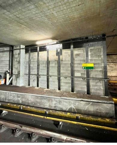
The upper 2' of the wall was confined with SRS-600UNI to to provide reinforcement where cracking had occurred. Additionally, 6" wide SRS-600UNI was installed vertically at 3' centers on both faces of the wall to increase the flexural strength and reinforce the wall against future failures.
