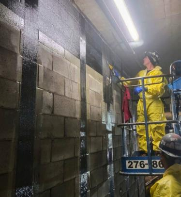
To address this challenge, Retro Specialty Contractors (Retro) reached out to SRS for help in developing a reinforcement plan for the wall utilizing Carbon Fiber Reinforced Polymer (CFRP).
