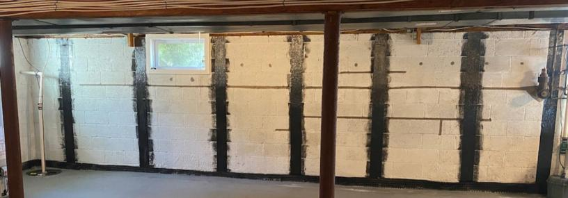
Excavating and pushing walls tends to be much more expensive and the access situations on the project do not always allow this. Additionally, if you are going to the expense of pushing the wall back, it's always a good idea to add reinforcement to keep the wall from bowing in again.
