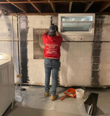
The tensile strength of the carbon fiber will resist any further inward movement of the wall, but into order to lock the wall in place, the mortar joints also need to be repaired as well. The best way to do this is the knock out the cracked mortar and completely re-tuck these joints.
