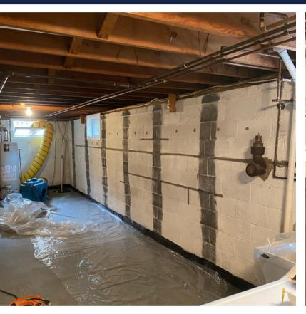
In bowed wall cases such as this, by using carbon fiber, contractors are able to provide homeowners a more cost effective solution to repair the wall and stop any further movement than possible with conventional methods.
