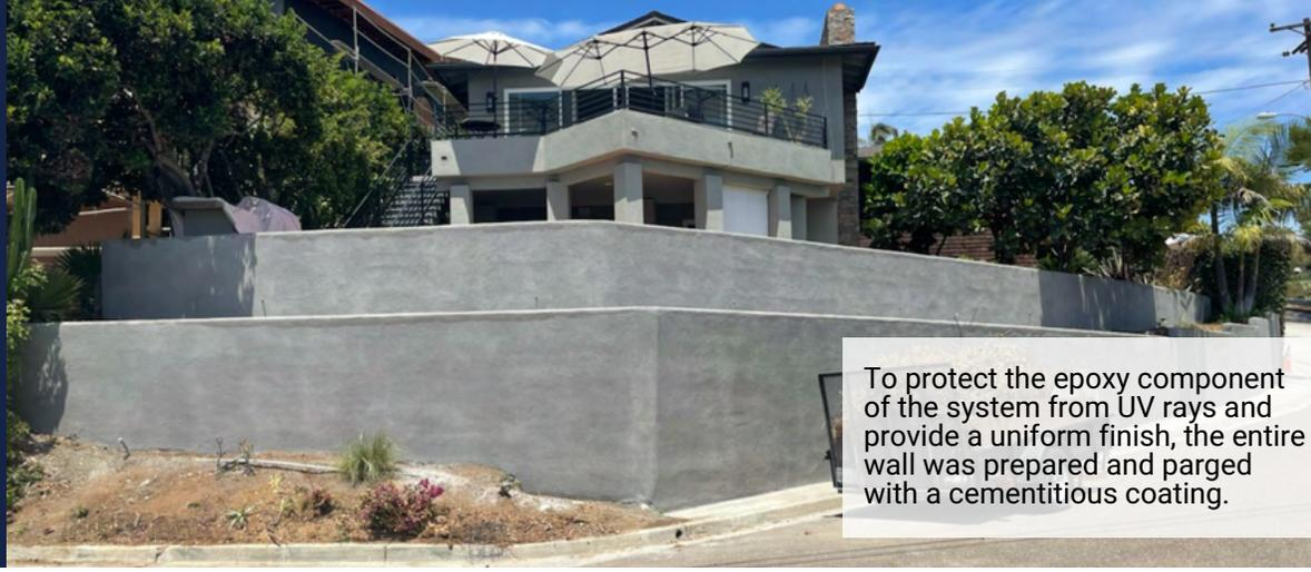
To protect the epoxy component of the system from UV rays and provide a uniform finish, the entire wall was prepared and parged with a cementitious coating.
