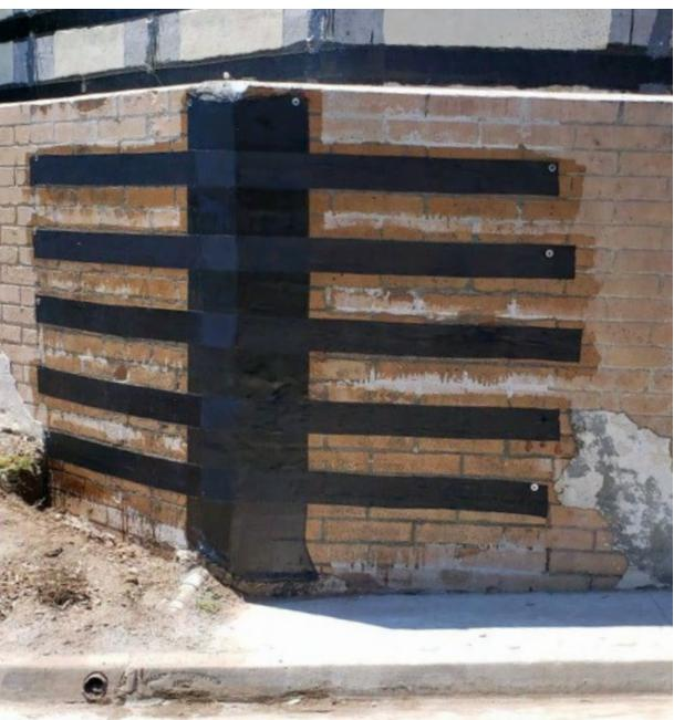
The surface of the bricks were prepared and cleaned prior to bonding the 24" SRS-660 bidirectional carbon fiber as a localized crack repair.
