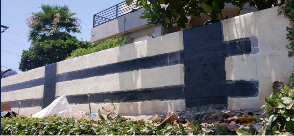
Due to the extremely high tensile strengths and very little elongation, the SRS-600 unidirectional carbon fiber is ideal to strengthen concrete structures such as columns, beams or walls. Providing design strengths over 196,000 PSI, this material delivers much greater reinforcement capabilities than steel, is non-corrosive, and at a fraction of the weight by comparison.
