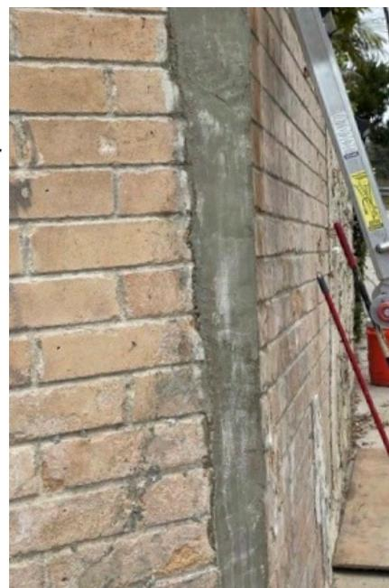
The large void in the broken corner joint was filled with a non-compressible hydraulic cement prior to the installation of the CFRP. To ensure a flat and even profile was met beneath the carbon fiber, each mortar joint was filled flush to allow for the SRS-600 Unidirectional carbon fiber to be securely wrapped around each side to provide global strengthening of the corner.
