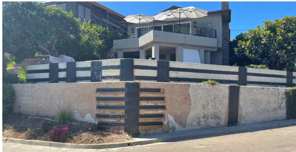
When concrete retaining walls fail, it can mean not only extensive landscape damage, but pose a significant safety risk to the public or surrounding property if left unaddressed. Retaining wall damage can be caused by saturated soils that result from improper drainage, footing damage due to settlement, rotation issues, or reinforcement deterioration over time.
