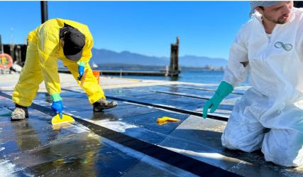
The layout of the carbon fiber was mapped out onto the concrete surface, which was prepared to achieve an optimum surface profile for carbon fiber embedment. This critical step ensures that any surface contaminants are removed, further opening the pores of the concrete to maximize the adhesion of the carbon fiber to the surface. Additionally, this light scarification of the concrete allows the ultra-thin CFRP (Carbon Fiber Reinforced Polymer) to lie flush with the surface.
