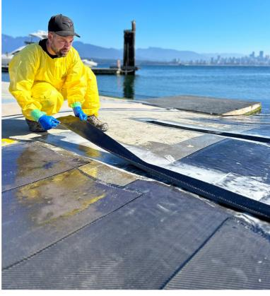
On day two of the installation 6" SRS-600UNI straps were applied to over the bidirectional to complete the global strengthening of the area and feathered into the previously installed CFRP to conceal the edges of the fabric.
