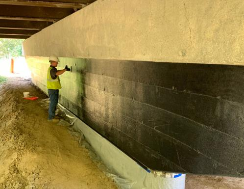
Epoxy injection was utilized to fill the vertical cracks using the SRS-1000 Structural Epoxy Resin in conjunction with the SRS-2000 Epoxy Paste to seal the cracks and set the injection ports.
