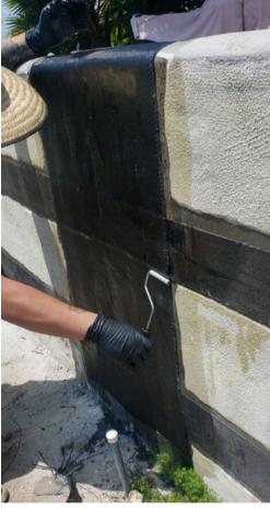
With a confinement strength of over 35,000lbs per sq/ft, the 24" SRS-660 Bidirectional carbon fiber extended up the outside face, across the top and down the inside face of the wall cracks.
