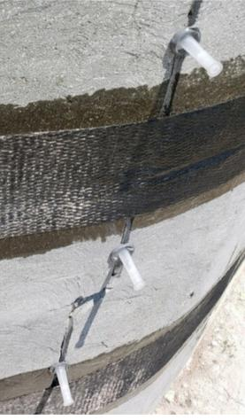
Injection ports were secured to both sides of the vertical cracks prior to them being injected with SRS-1000 Structural Epoxy Resin. The high strength non-compressible resin was used to fill the voids and bond both sides of the wall together at the crack locations.
