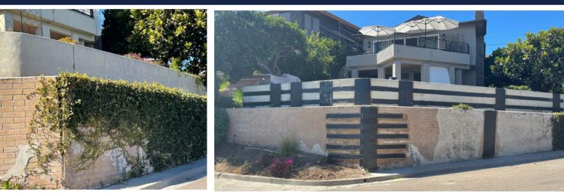
When concrete retaining walls fail, it can mean not only extensive landscape damage, but pose a significant safety risk to the public or surrounding property if left unaddressed. Retaining wall damage can be caused by saturated soils that result from improper drainage, footing damage due to settlement, rotation issues, or reinforcement deterioration over time.
